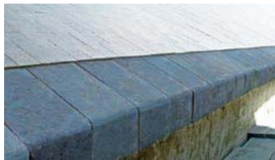
A coke ramp protected by KALMETALL®-C in combination with silicon carbide ceramics KALSICA® and hard ceramics KALCERAM®-K.
