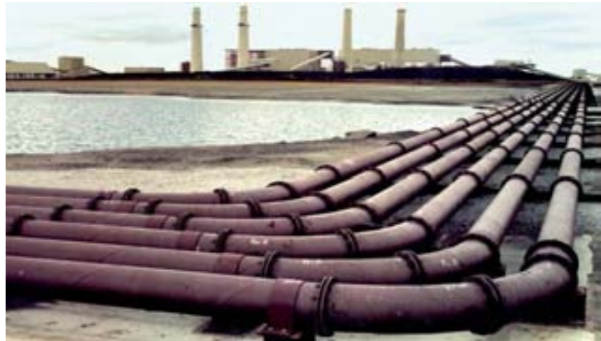
Wet ash pipe in North America; the pipes are flanged together
