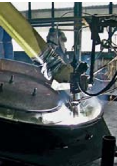
Service by Kalenborn: rebuilding a grinding table with KALMETALL-W 100
