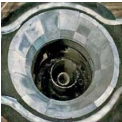
Reflectors of PF-burners protected by KALSICA-N (photo) or KALMETALL-W
