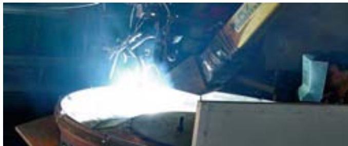
Kalenborn supply wear protected plant components. In addition we provide for regeneration of worn components - here a grinding table of a coal pulverizer.
