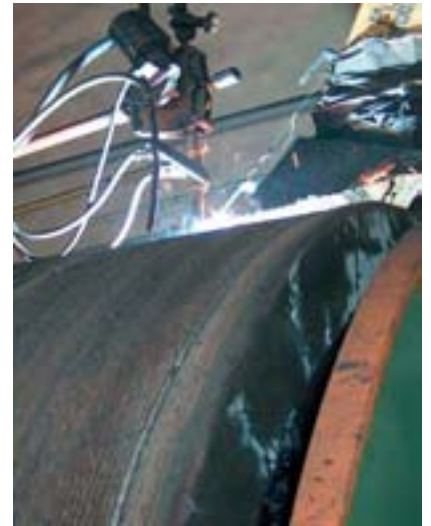
Kalenborn Service solves wear problems on site
