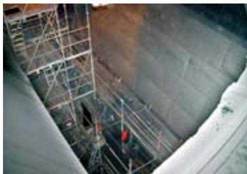
Coal bunkers lined with KALEN slide promotion plastics ensure a reliable material flow
