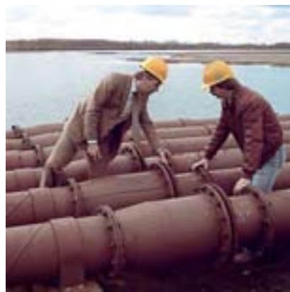
Long pipes require the use of expansion joints for compensation of length
