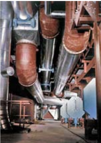
A typical application in power plants is pulverized fuel piping, here protected by ABRESIST
