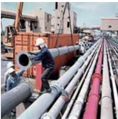
Erection of wet ash pipes in Malaysia (350 mm diameter)
