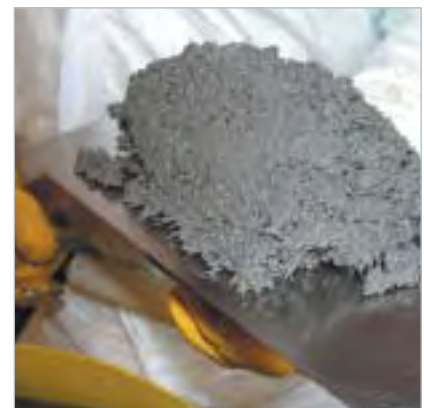
6. The stiff/plastic KALCRET compound (X) to be applied by trowelling is compacted with the aid of a vibration trowel
