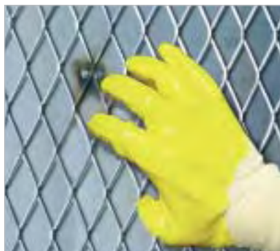
Stiff and rigid fastening – distance to the wall to be lined: about 5 mm
