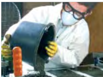
3. Carefully fill formwork
