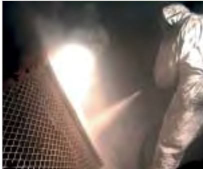
KALCRET spraying technology
