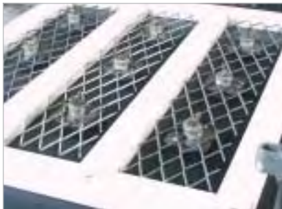
1. Prepare formwork
