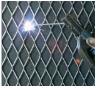
Welding the wire mesh to the surface to be lined: distance approximately 250 mm
