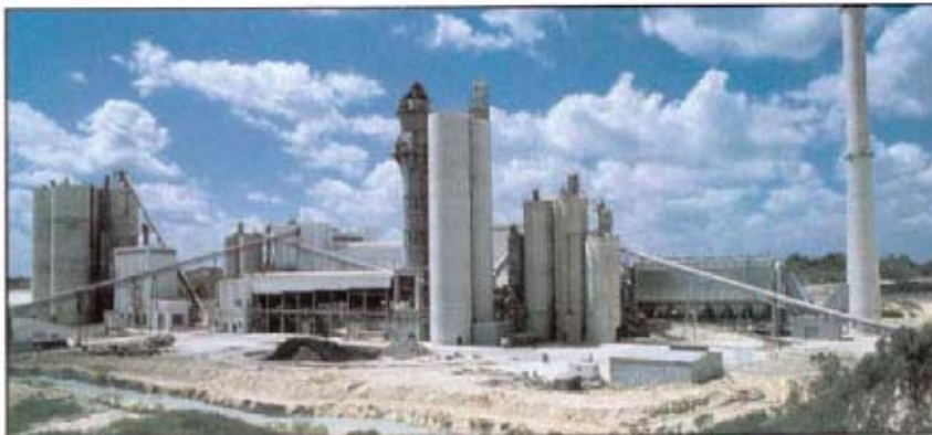
Florida Crushed Stone's Brooksville cement plant processes 600,000 st/y of Type I and Type II portland cement.
